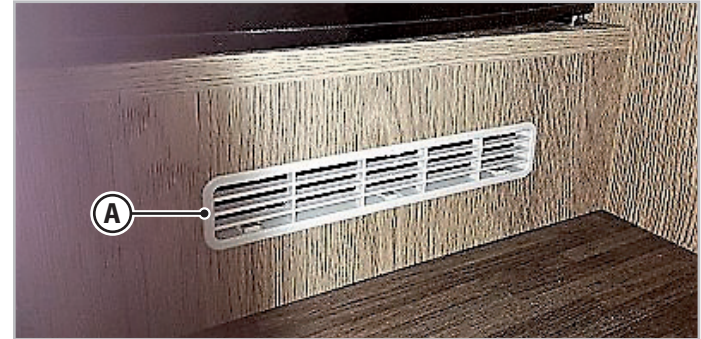
Fig. 6.1 - Permanent ventilation openings
